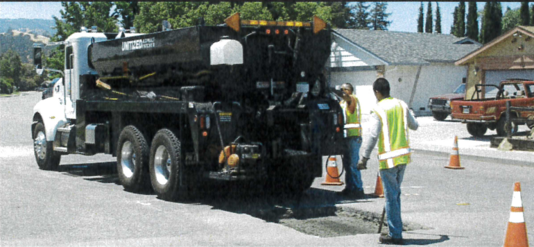
Remove old material, create a firm base and tack the hole edges.
